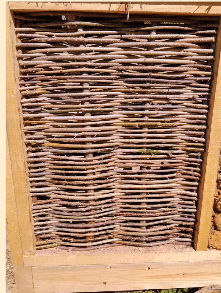
Cebatu with horizontal branches that are placed on top of each other
