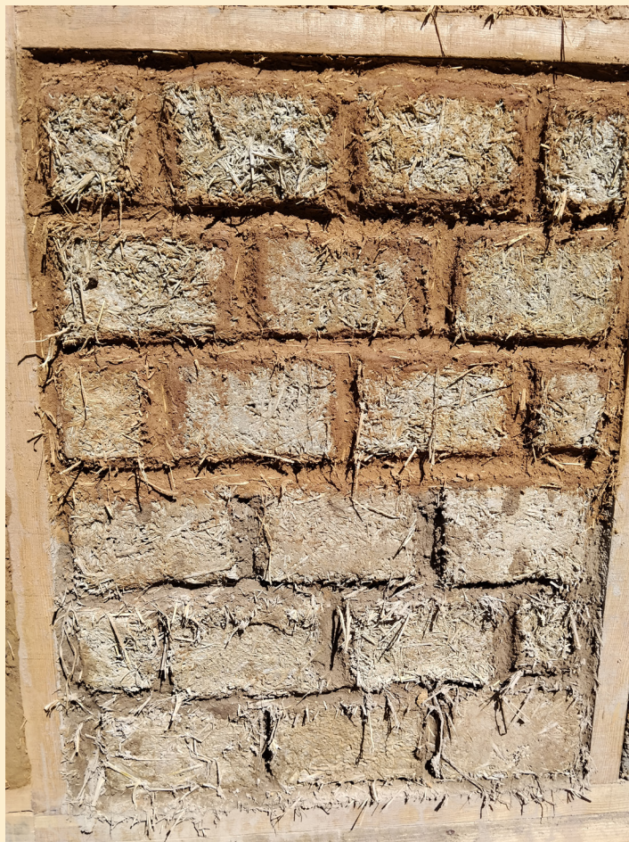
Finished wall from Adobe bricks
