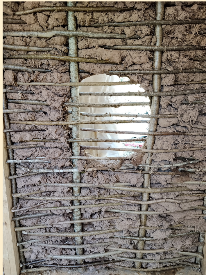
Cebatu with horizontal branches placed with spacing
