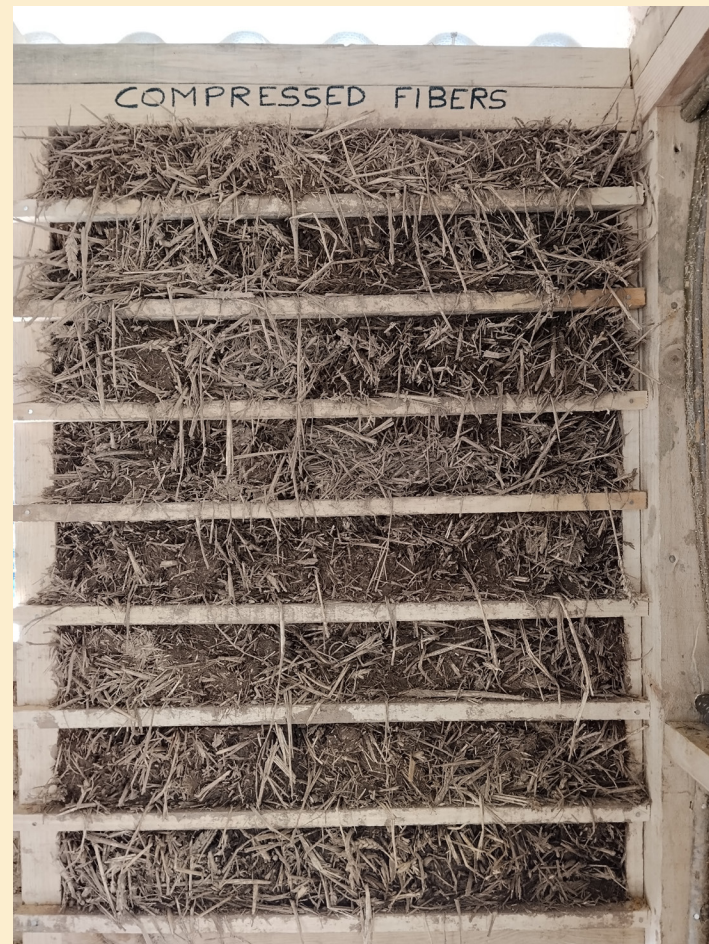
Light clay with slats and long straw
