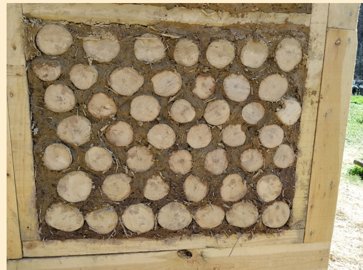
Cordwood wall from outside
