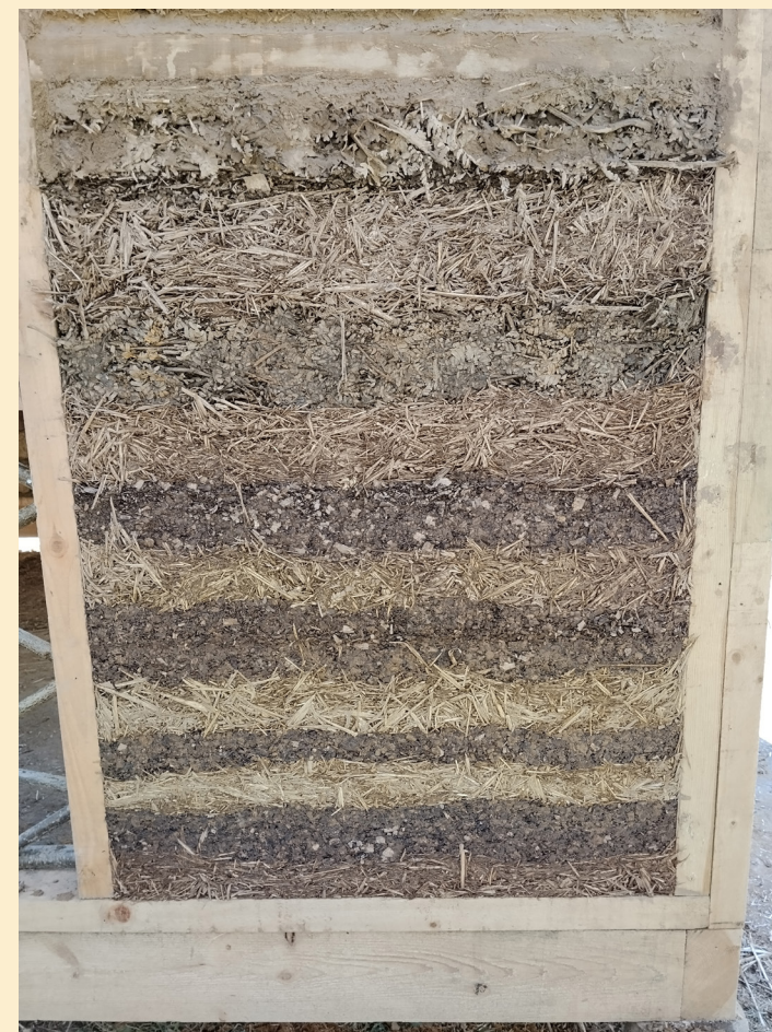
Light clay with layers of wood chips, long straw and fern
