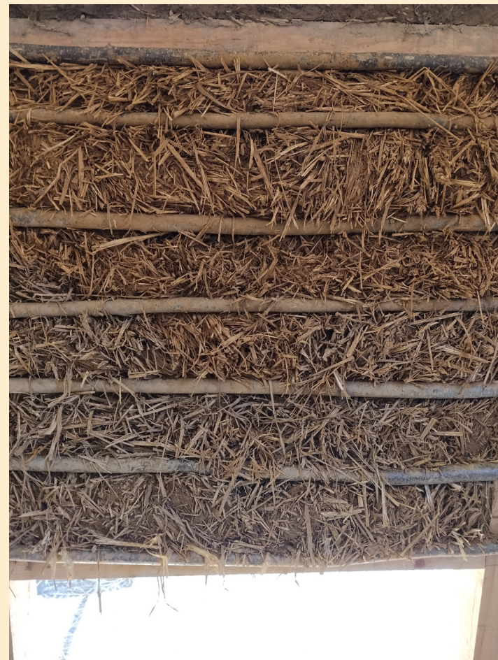
Light clay with slats and long straw
