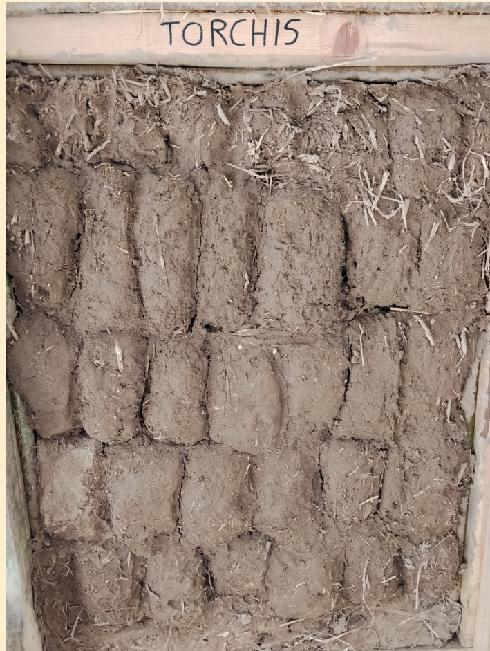
Loaves that are hung in a loop on the horizontal battens
