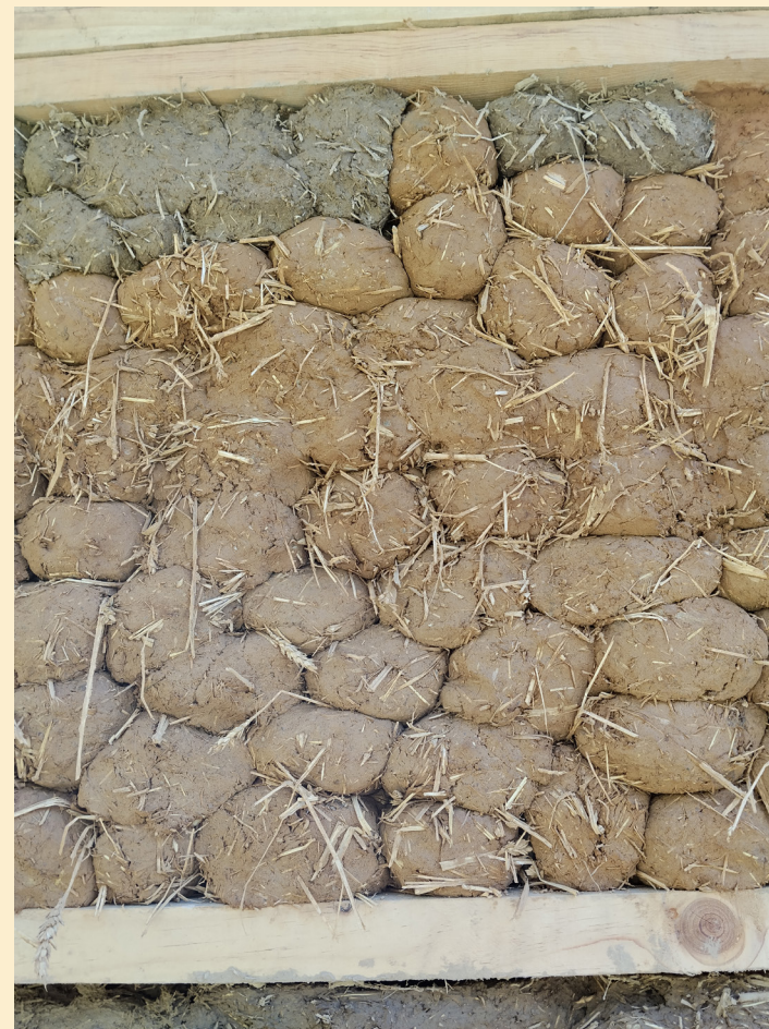
Cob in form of balls placed on each other
