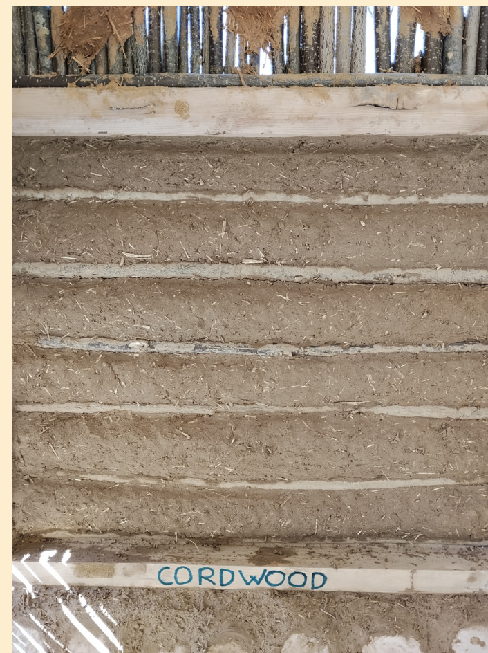
Light clay with slats and long straw
