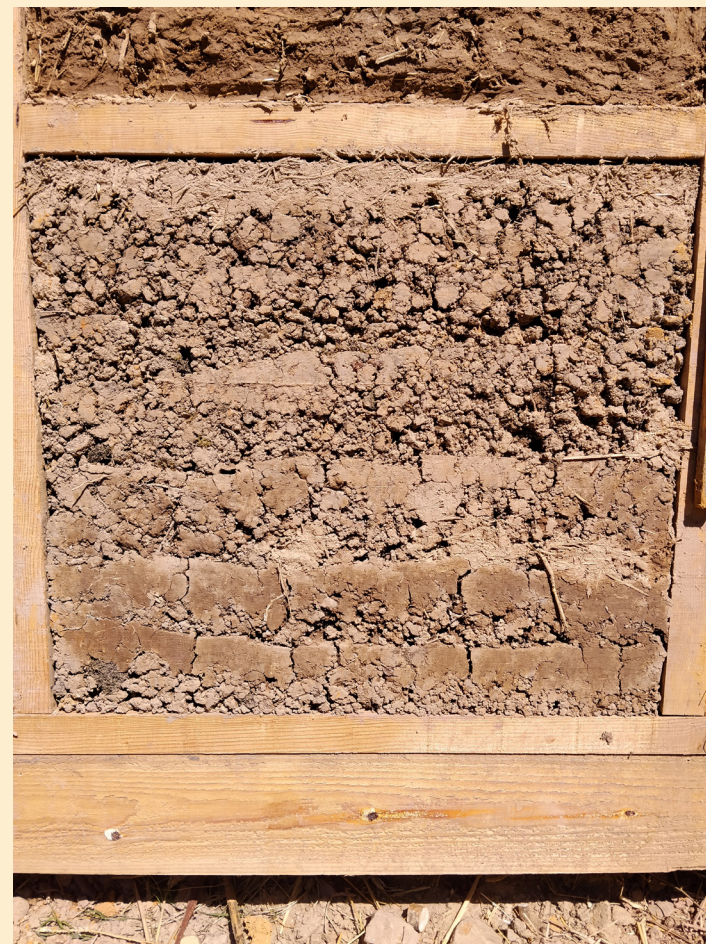
Rammed earth with clay that has lighter color
