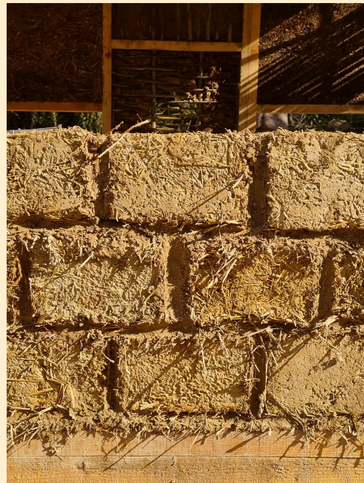
Detail on Adobe bricks during construction
